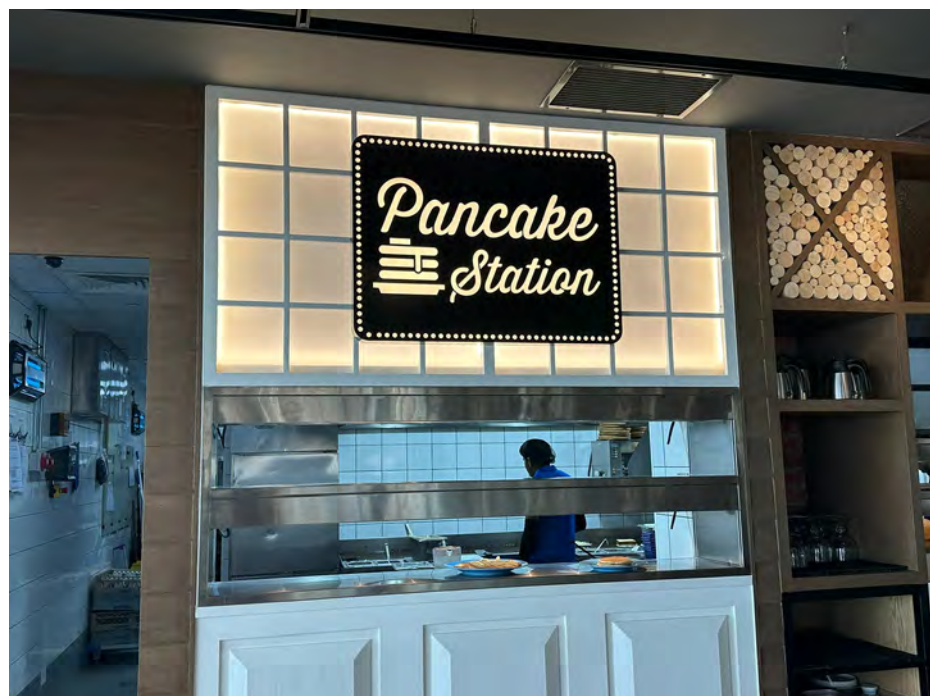
Aluminum powder coated with stencil cut and install on the existing backing with light
