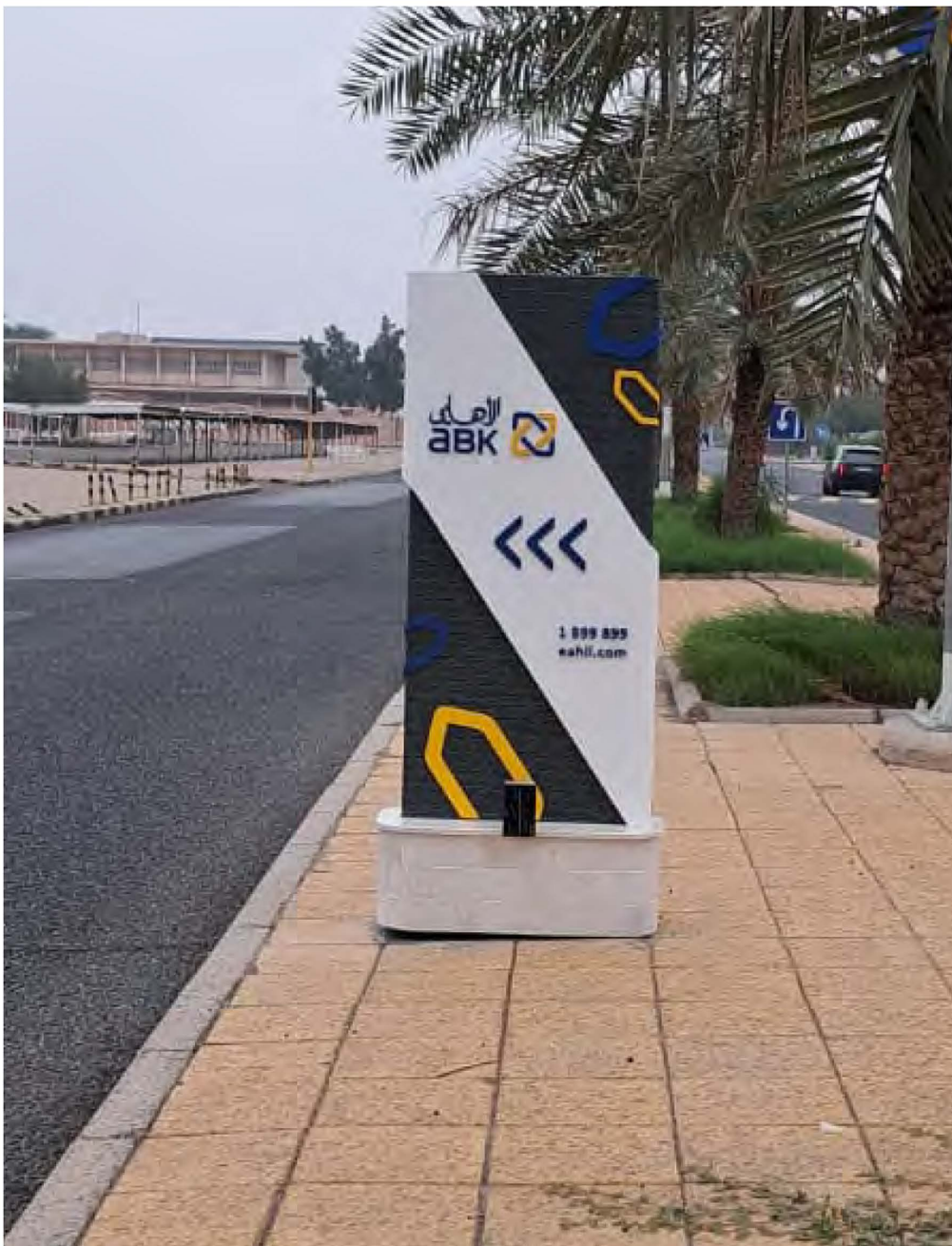
Road Signs made of Heavy Duty base plate with concrete base All perforated sheet bend and shaped to match two sides and powder coated along with aluminum laser cut with white powder coated, installed with acrylic bend and shaped to match the design
